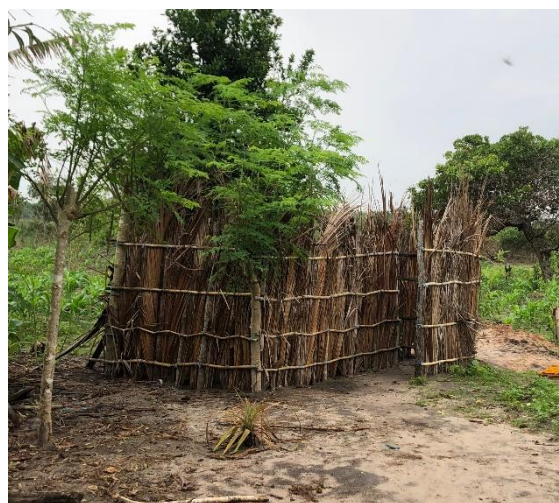
Photo : Simple pit latrine in Namala 2
