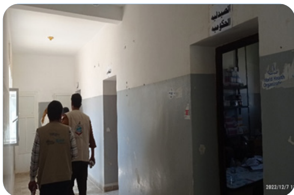
Figure 5 the hospital interior condition
