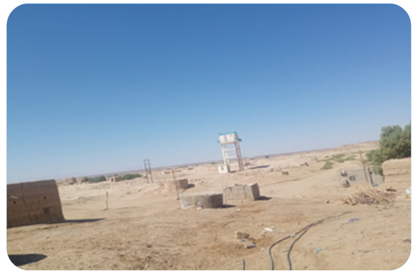
Figure 4 water supply tanks that not functioning or supplying the community
