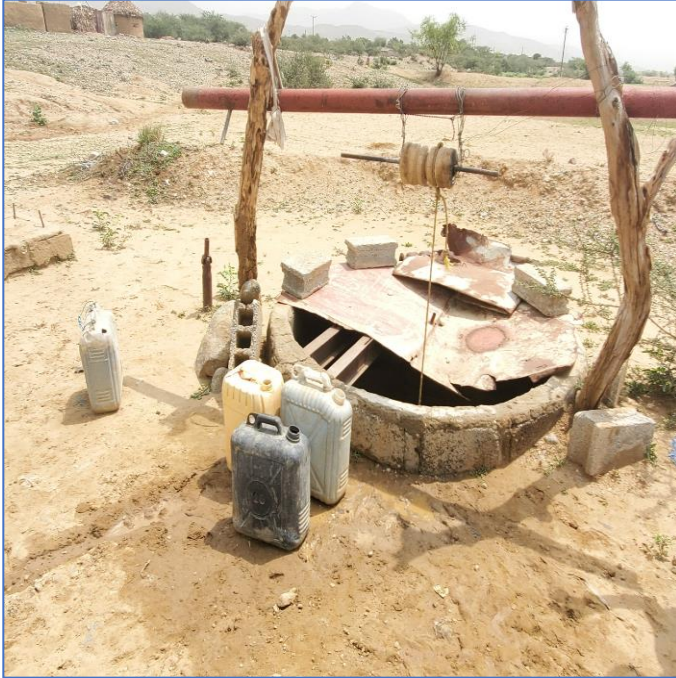
Photo 5 Unprotected Well exposed to contamination - Al Hamur IDPs site - Sep 6, 2022
