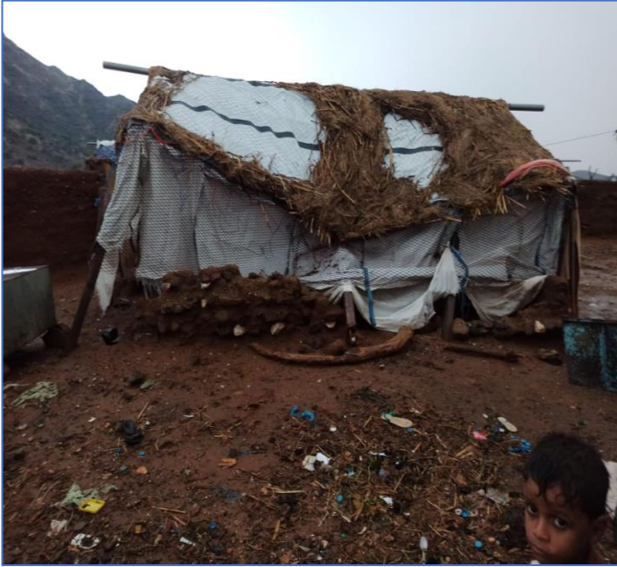
Photo 1 Destroyed Shelter by heavy rain - Al Dabayah IDPs site – Sep 04, 2022
