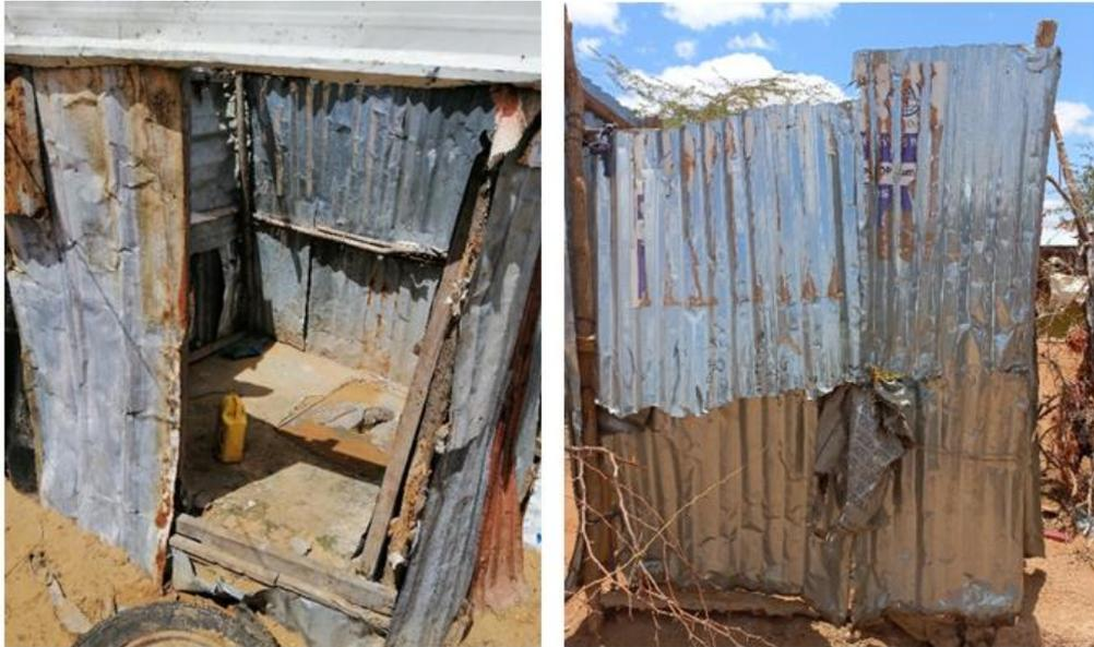
FIGURE 1: LATRINE WITH MISSING DOOR IN BANADIR (LEFT) AND A BROKEN LATRINE SUPERSTRUCTURE IN DOLLOW (RIGHT) PHOTO COURTESY SSWC/CRS
