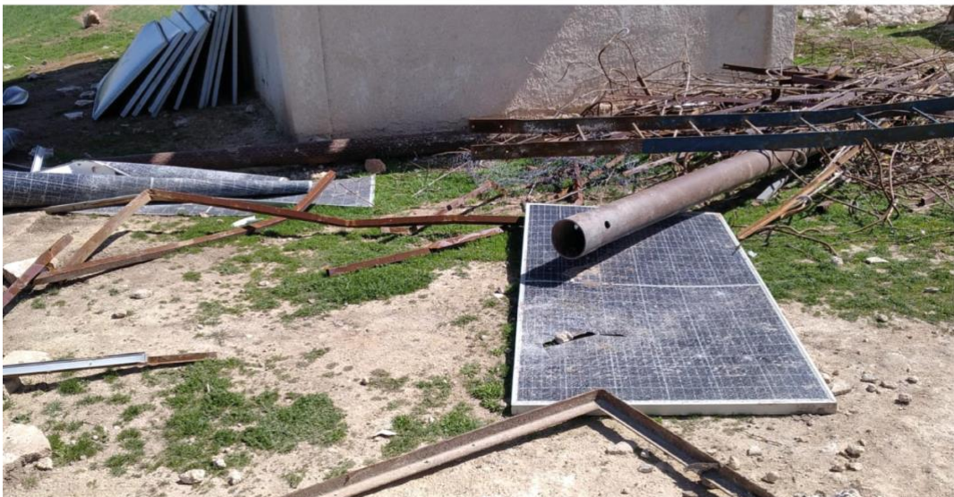
Damage to irrigation infrastructure, March 2023. ©FAO.
