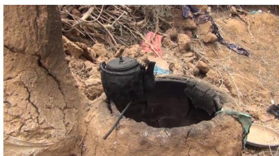
Flood-damaged, improvised kitchen.
