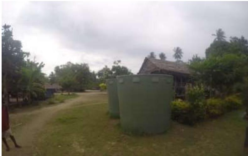
*Figure 4. 2 x 9000L water tanks distributed by the District Administration in late 2015. These are typical of those found on all the islands. With only one or two exceptions where local materials have been used to connect the tanks to existing roofs, these tanks are unused as they were delivered without fittings.*
